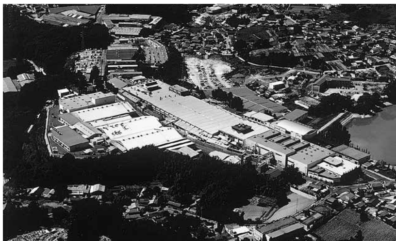
KITZ Nagasaka Plant, Japan
